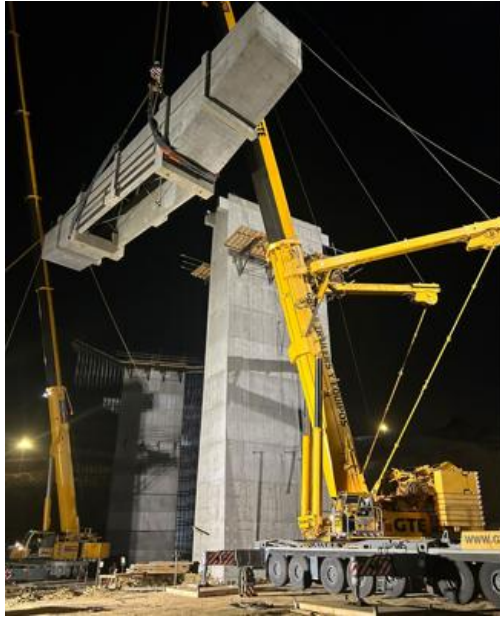
Fig. 1. Precast pier caps of the Matadero Viaduct in Tijuana (México).
