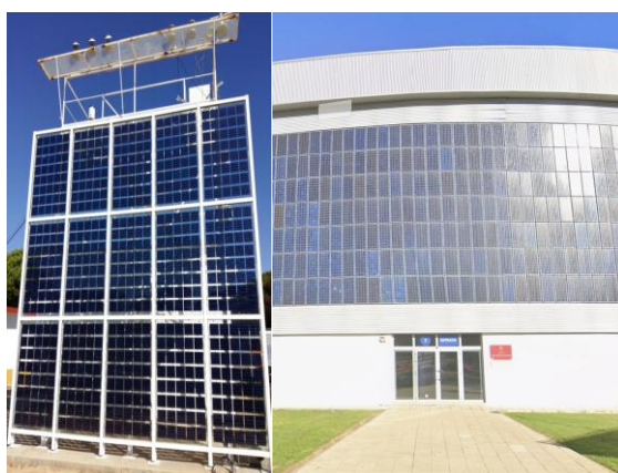
Fig. 1. Vertical PV integrated for building integration. INTA and University of Huelva.
