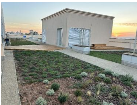
Figure 1. Example of extensive green roof in Lleida. Agrobiotech Park (Lleida, Catalonia, Spain)
