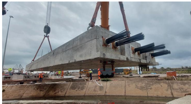
Fig. 2. Precast slab of the Arcelor Canal Bridge in Sagunto (Spain).
